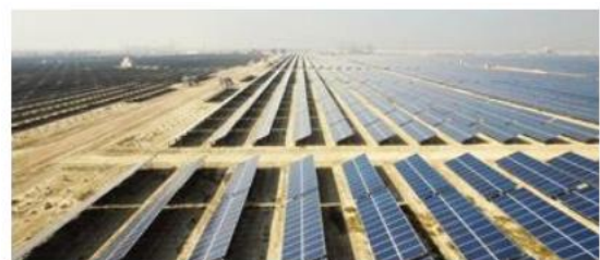
Fig. 1. Quaid-e-Azam Solar Park at Bahawalpur 1000 MW capacity
